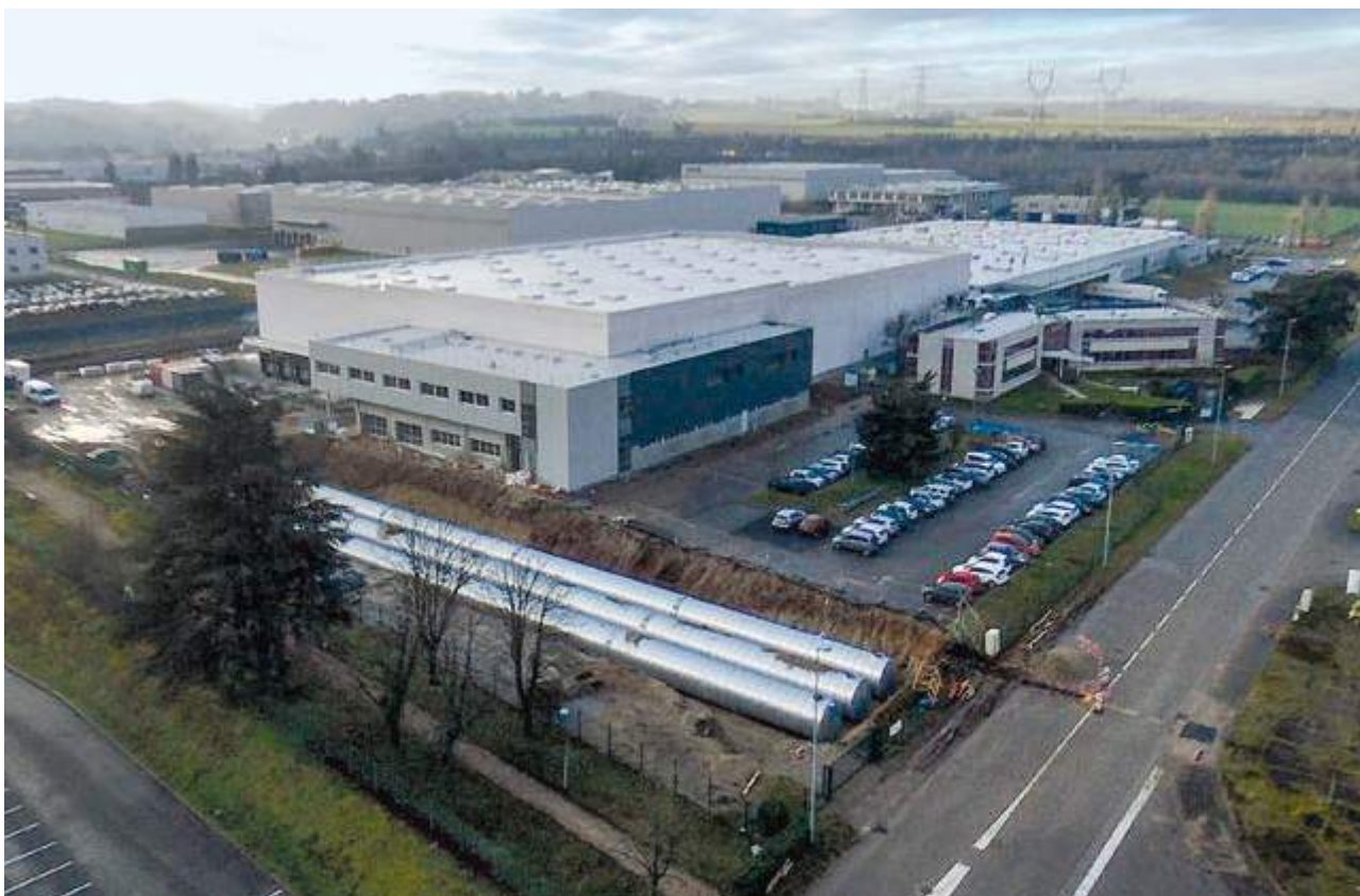
Dipra's underground water retention system.
