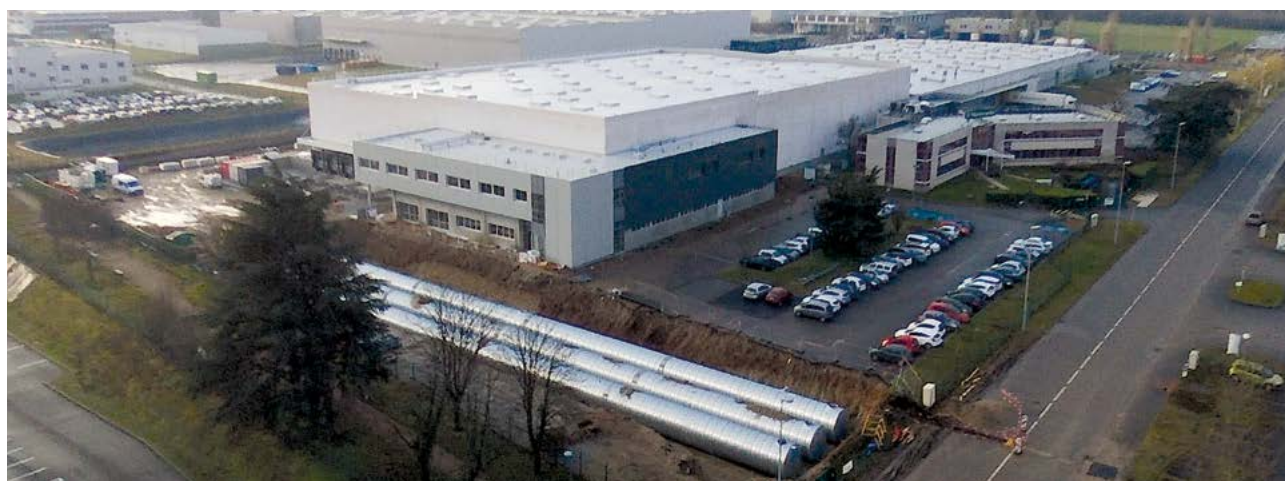
The new Dipra building is also equipped with a rainwater recovery system.
