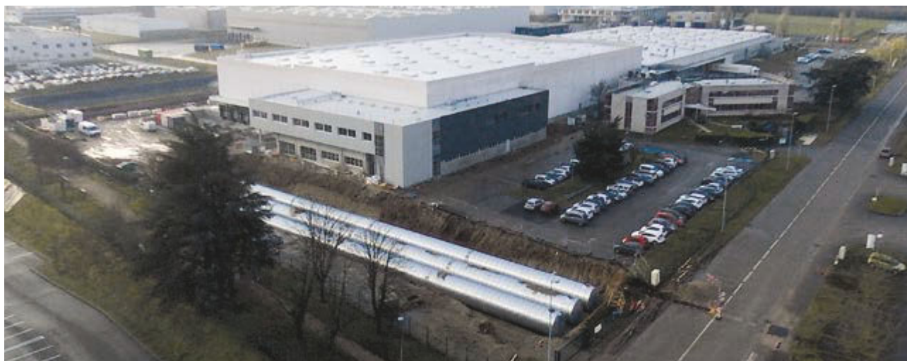
The new Dipra building will also be fitted with a rainwater recovery system
