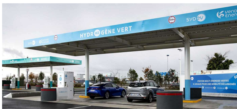
Green hydrogen station in Roche-sur-Yon (Vendée) powered by hydrogen produced by Lhyfe
