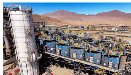
Chile: Mantoverde Mine
