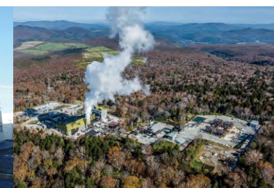
Appi Geothermal Power Plant
