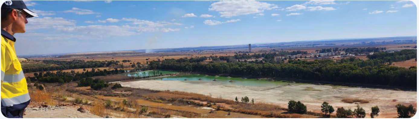
Driefontein engineer of record tailings dam audit, Carletonville, South Africa, downstream view
