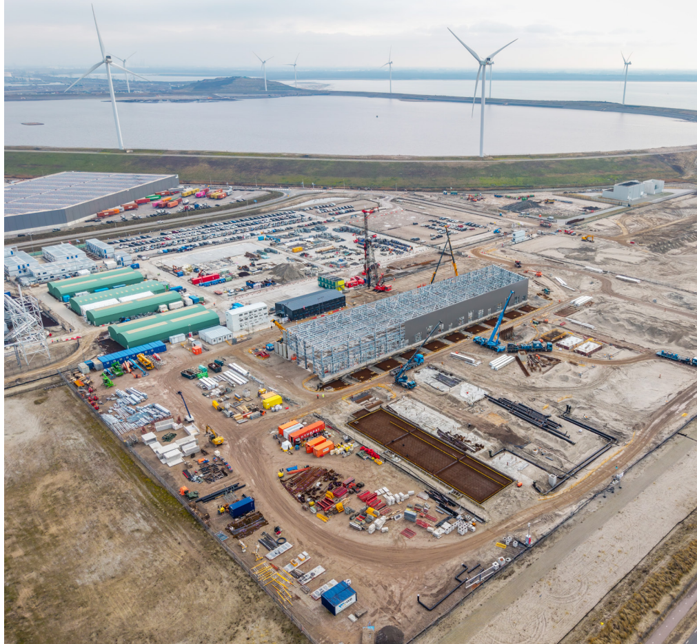
● ELYgator electrolyzer construction site, in Maasvlakte, the Netherlands.
