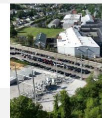
Jeannette Power Facilities
