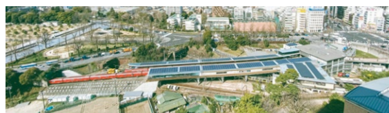
Solar power generation systems
