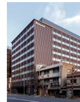
OVOL Kyoto Ekimae Building
