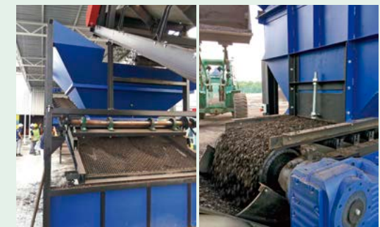
PKS being loaded into a receiving hopper by heavy machinery
