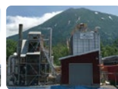
2017 Corelex Doh-Ei Introduction of a biomass boiler
