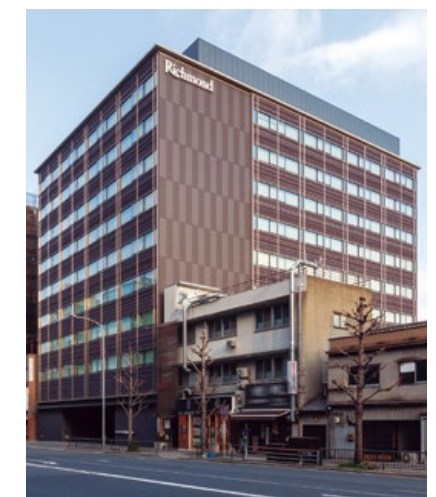
OVOL Kyoto Ekimae Building
