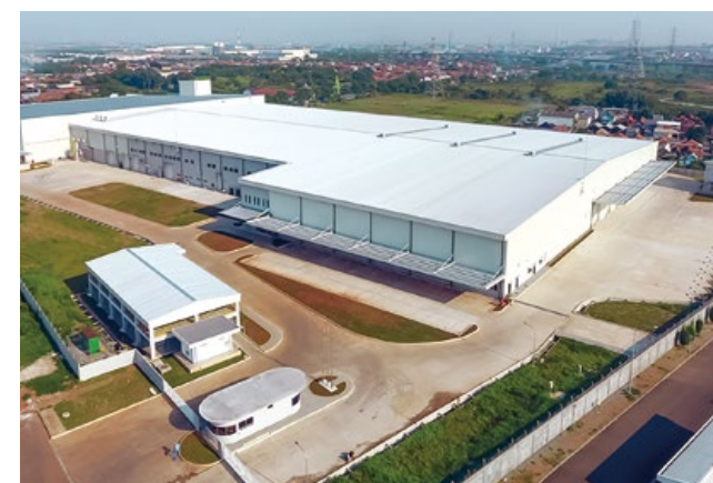
Panoramic view of the new plant
