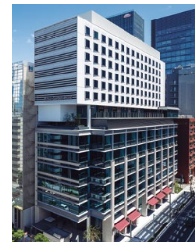
OVOL Nihonbashi Building
