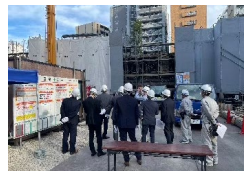
▲Safety patrols by the Building Subcommittee [New condominium construction site] (Checking the scaffolding and crane operations)
