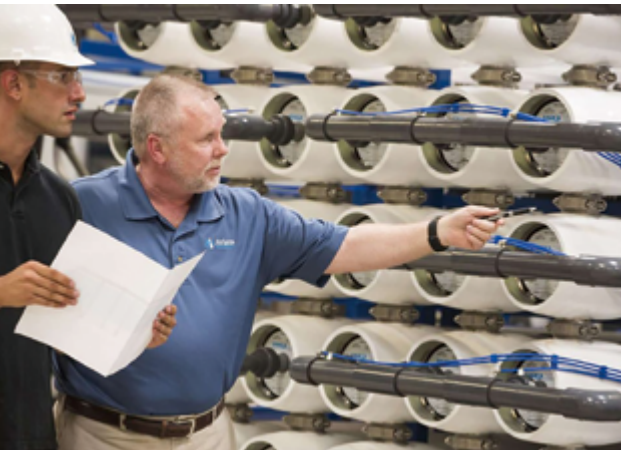
Image of RO membranes
