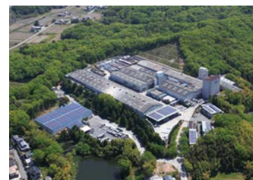
Hyogo Factory mega solar
