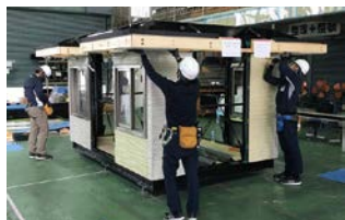
Framing/exterior course: completion test
