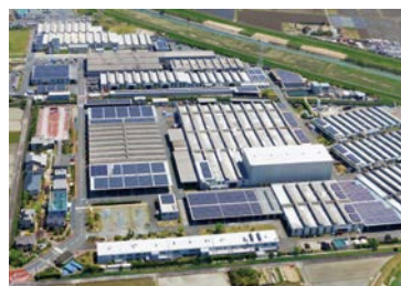
Shizuoka Factory mega solar
