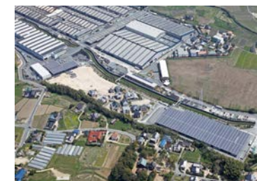
Yamaguchi Factory mega solar
